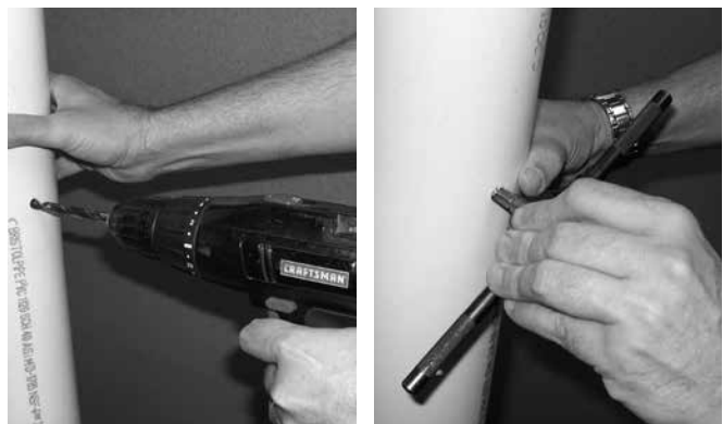
Figure 9.1: Drill and Tap Combustion Test Port
