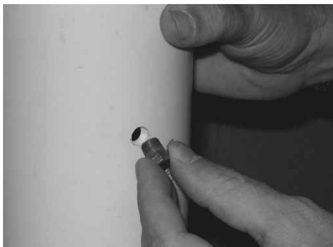
Figure 9.3: Insert Pipe Plug into Test Port
